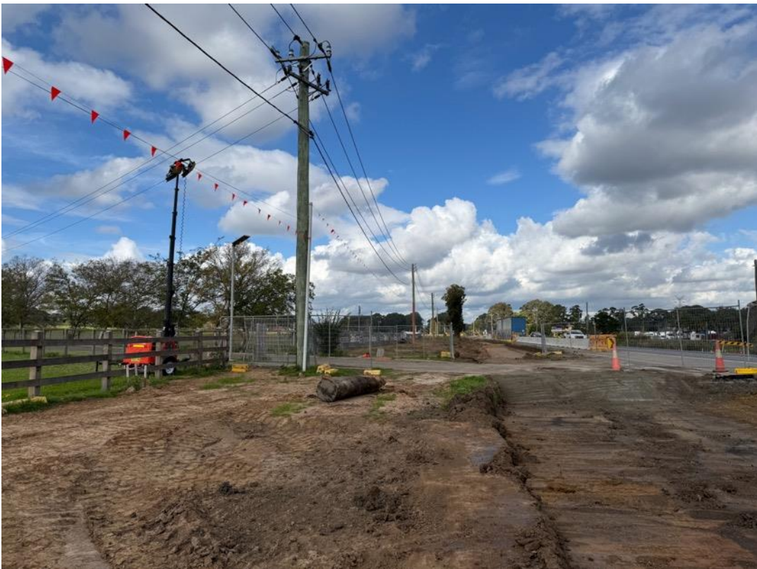
Plate 8: Neighbours driveway. Note the presence of ongoing access and the lights to enable safe entry/ exit for the resident. (South of Abbots Road)
