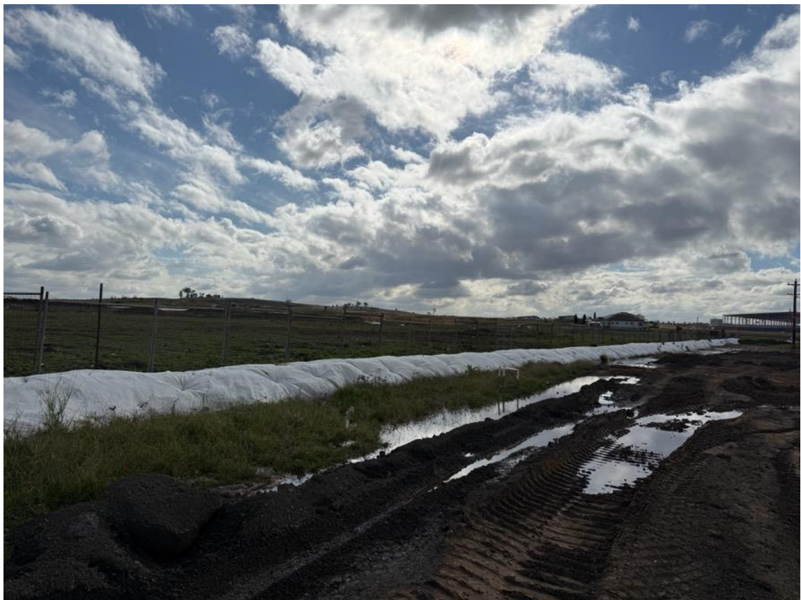
Plate 12: Boundary erosion and sediment controls in place.
