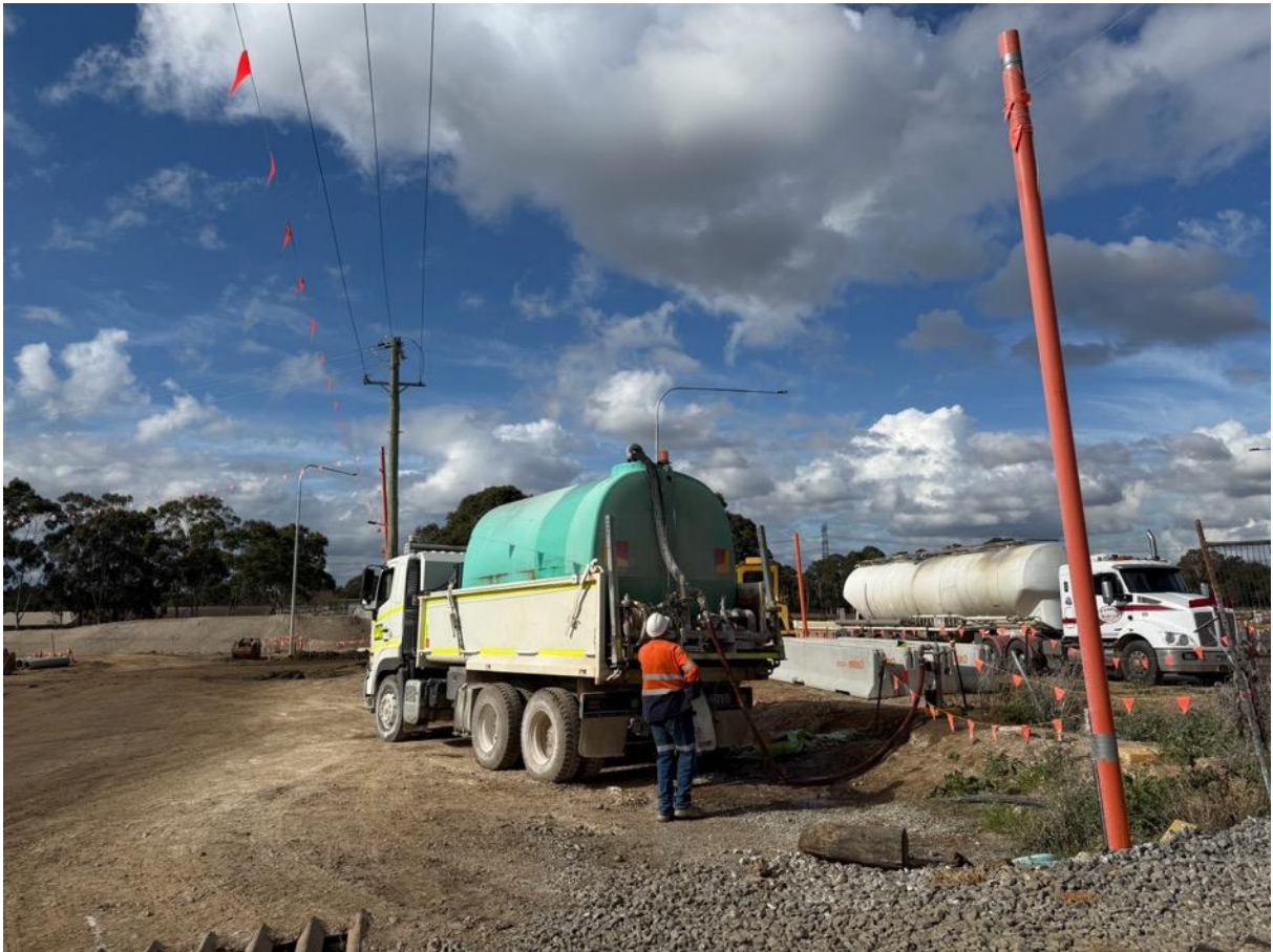
Plate 11: Water truck refilling on site. There were no visible dust plumes from the project during the inspection.
