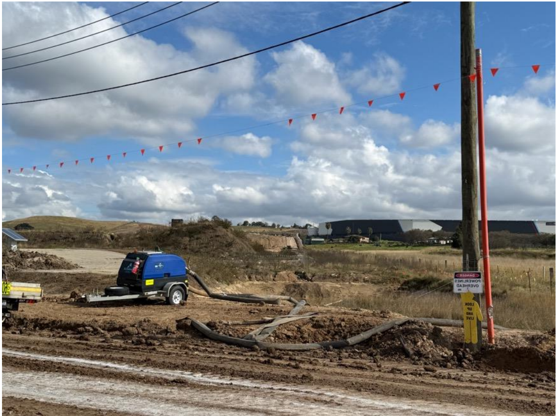
Plate 5: Water reuse from decommissioned dam. (South of Abbotts Road)
