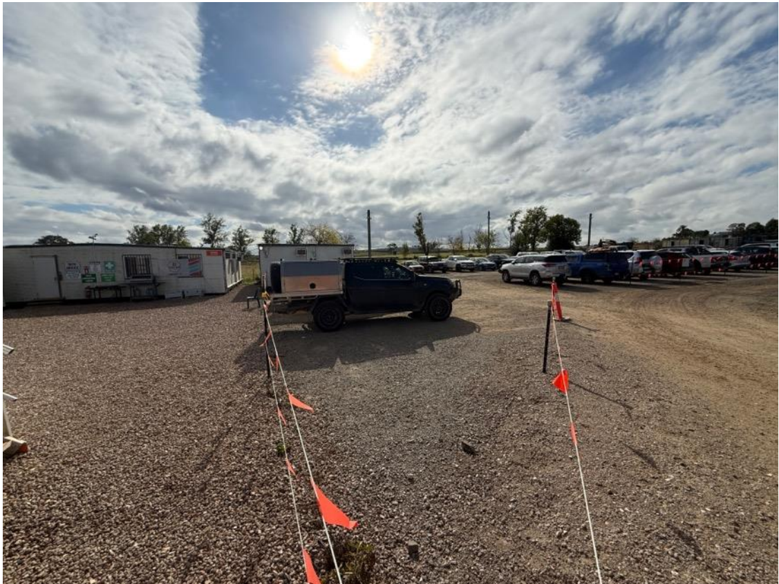
Plate 1: Light vehicle parking, pedestrian separation and heavy vehicles in the back.
