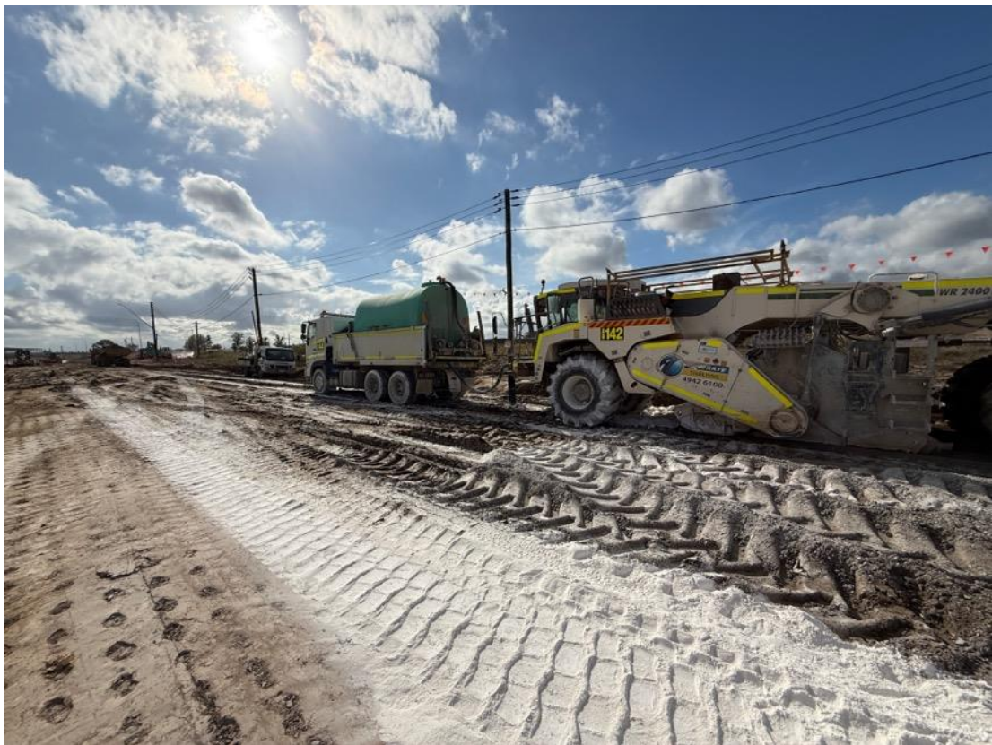
Plate 4: Water cart and machinery involved in the lime application. (South of Abbotts Road)
