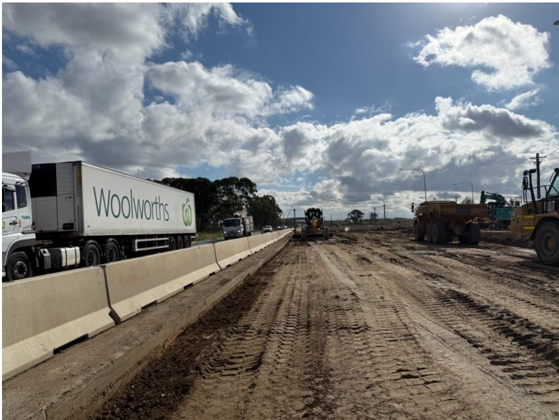
Plate 6: General site works and traffic barriers. Mamre Road is a high traffic road, that has necessitated some out of hours works. (South of Abbotts Road)
