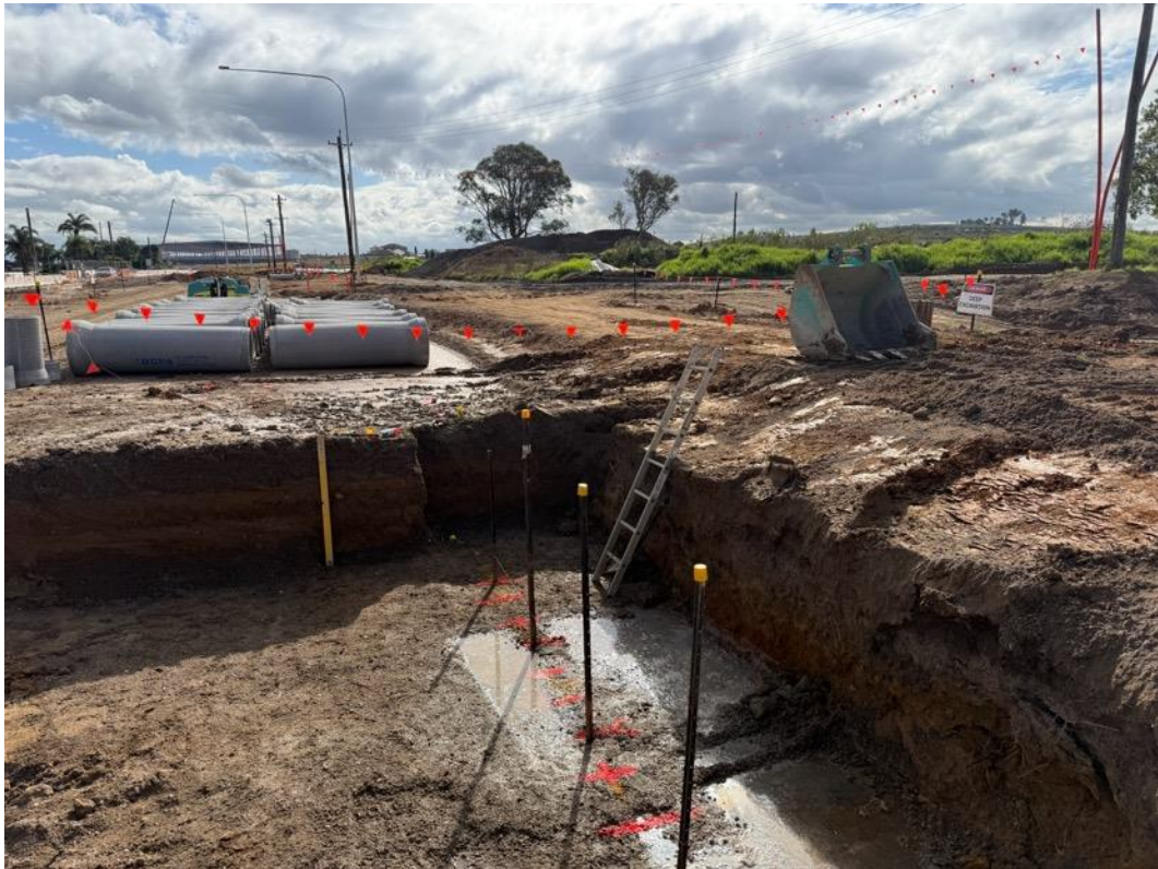
Plate 9: Excavation and stormwater infrastructure (North of Abbots Road)
