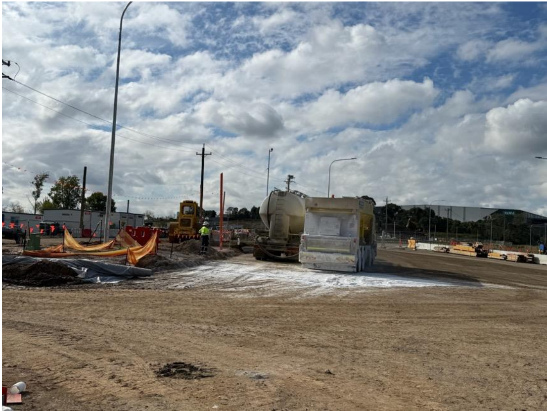
Plate 3: Bulk loading of lime into equipment for material stabilization treatment. (On Northern side of Abbotts Road)
